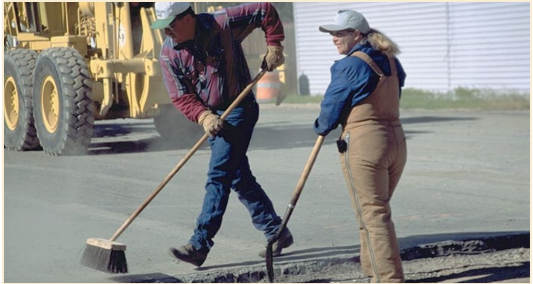
ACHD manages the planning, construction and maintenance of county roads.
